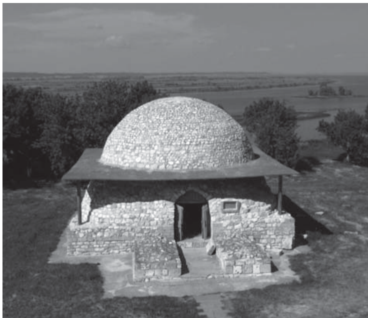
The Northern Mausoleum in the ruins of the fortified medieval city of Bulgar; built in the mid-14th century, it overlooks the Volga river. This structure now houses a collection of Islamic tombstones from the territory of the Volga Bulgar state; the rectangular modern roof protects the masonry from the severe weather characteristic of this region. (Photo V. Shpakovsky)
